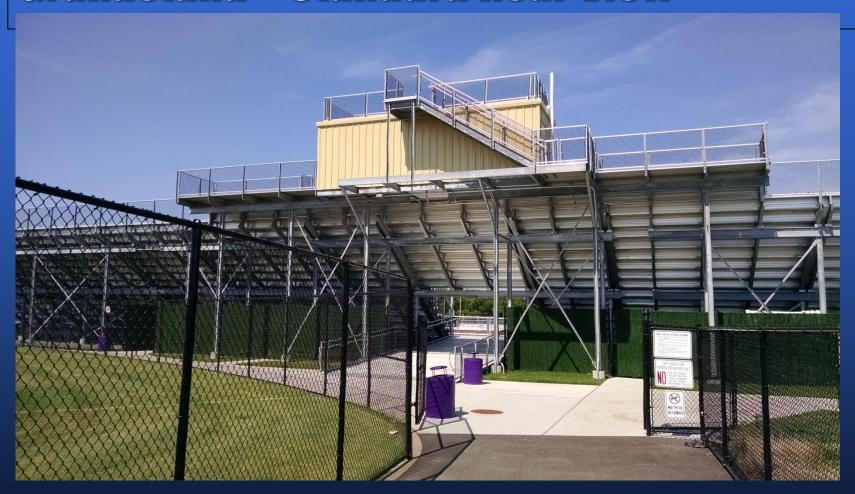
The standard rear view of Grandstand bleachers assembly. Exposed structure with chain link fence surrounds with privacy slats, flanking the vomitory entrances up into the stadium area. This is provided within the current bond
