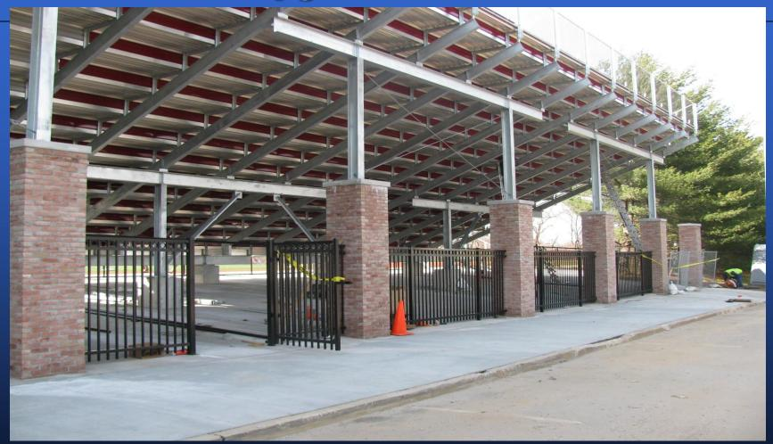
An upgrading of the standard exposed column treatment, rear view of Grandstand bleachers assembly. While an additional cost, the inclusion of brick pier surrounds and precast stone caps provide an upgraded style to the columns. Additional treatment can also include wrought iron fencing in lieu of black vinyl chain link fencing.
